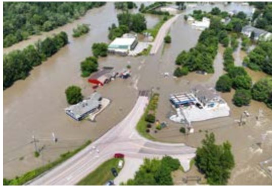
The village of Jeffersonville, VT, under water after the July 2023 floods. Photo: AJ Murray Photography
